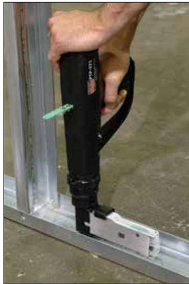
Rotating magazine allows for installation flexibility
