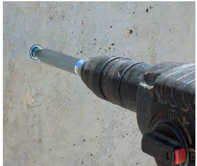
Anchor being set with SDS setting tool.
