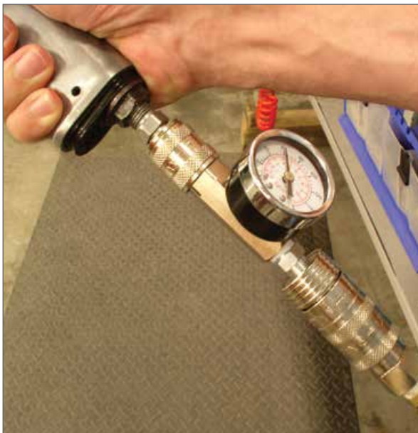
Testing pressure drop at the tool with a differential pressure indicator
