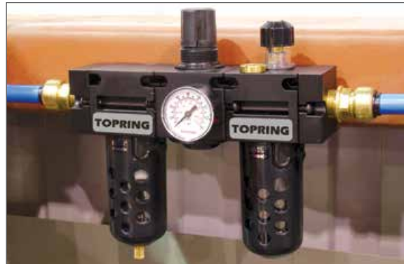
MODULAIR FRL with pipe adapters make for a very neat installation
