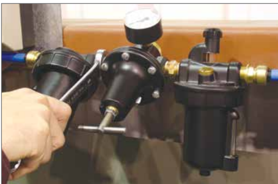
This makes maintenance very difficult
