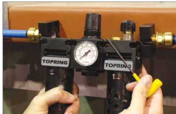
Removal is very easy, since the piping adapters allow the unit to slide out
