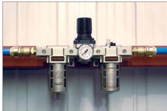
Modular FRLs with pipe adapters make for a very neat installation
