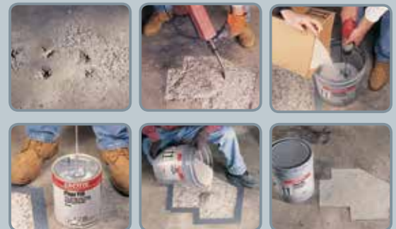
Your Source for FLOOR FILL Loctite® Fixmaster® Floor Fill 6-Step Process
